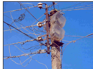
Figure 2.2 Insulated line for control of theft Figure 2.3 Pole with meter (to stop theft)
