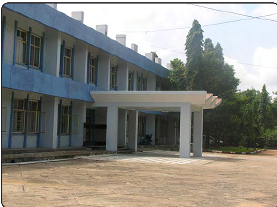
Photo-6: CIRE- Another view of Existing Administrative Building
