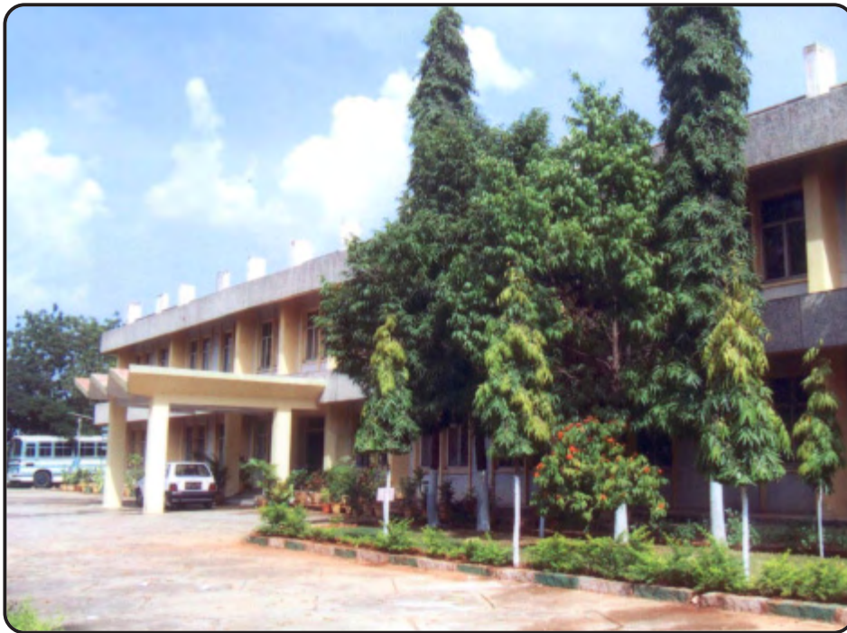
Photo-5: CIRE- Existing Administrative Building
